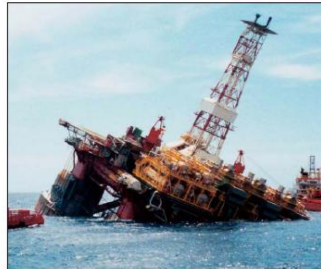
Figure 1: Petrobras P-36 sinks into the Atlantic Ocean.
